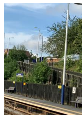
Limited coverage of CCTV
